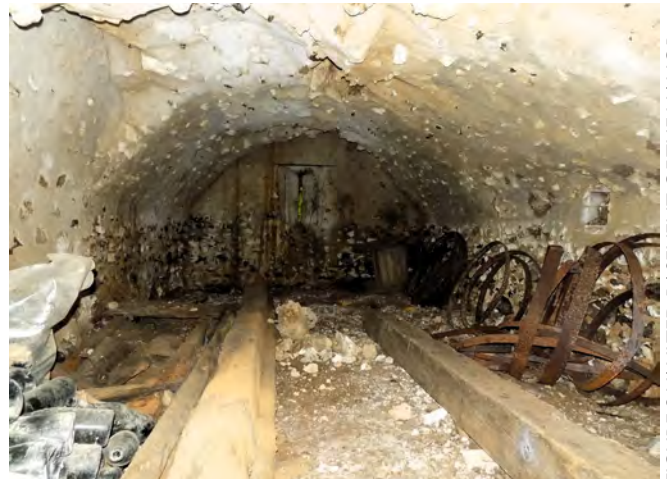
FIGURE 3: VAULTED BASEMENT OF THE MANOR STANDING IN THE EASTERN CORNER OF THE INTERIOR
