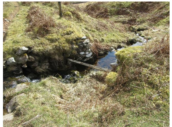
The abutment of a bridge over the Clinchie Cleuch Burn.
